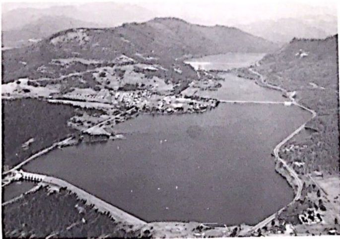
Figure 1-1. Dexter Lake is one of 13 multi-purpose water resource projects built and operated by the U.S. Army Corps of Engineers in the Willamette Valley. In combination with Lookout Point Lake and dam immediately upstream, it was completed in 1954 and provides flood control, hydroelectric power generation, and summer recreation. (Photo credit: U.S. Army Corps of Engineers)
